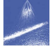
Rain curtains are installed to prevent fires spreading and to divide large spaces into fire sections as well as to shield wall, door and window openings.
