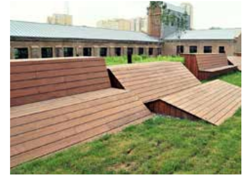
Reconstruction of Jilin Waterworks
