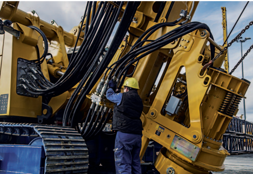
Rigging position for connecting of hydraulic hoses
