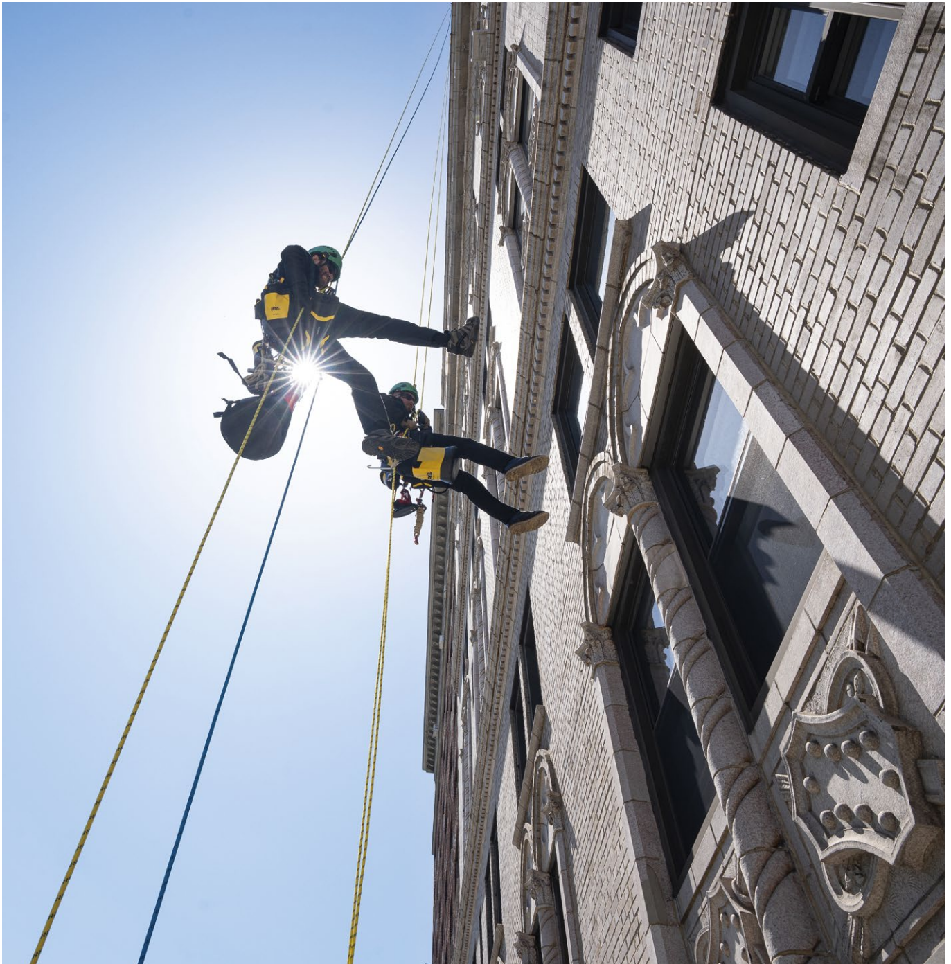
Historical building maintenance and repair, Central Park, New York City, New York, USA © 2024 Petzl Distribution - Vuedici.org - SPAR
